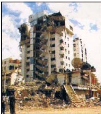
Fig. 3.3a: Destruction caused by an Earthquake at Bhuj
