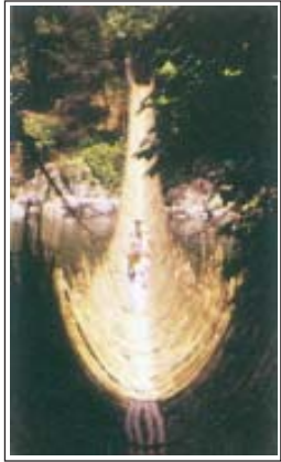
Figure 6.7 : Rope Bridge (Arunachal Pradesh)
