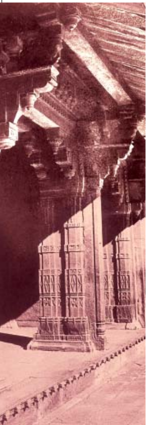
Fig. 17 Decorated pillars and struts holding the extension of the roof in Jodh Bai palace in Fatehpur Sikri. These follow architectural traditions of the Gujarat region.
